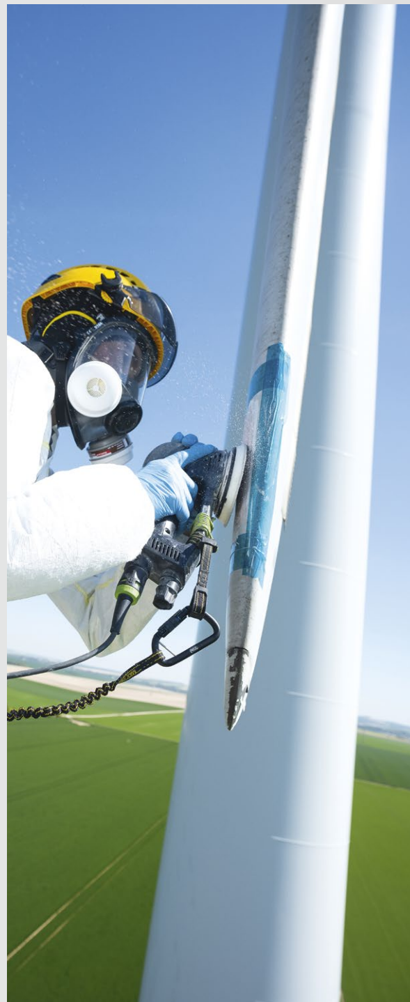
Wind turbine maintenance © 2022 Petzl Distribution - Vuedici.org - GR Wind - Vestas - Joly - EDF Renewables - Les Coteaux wind farm
