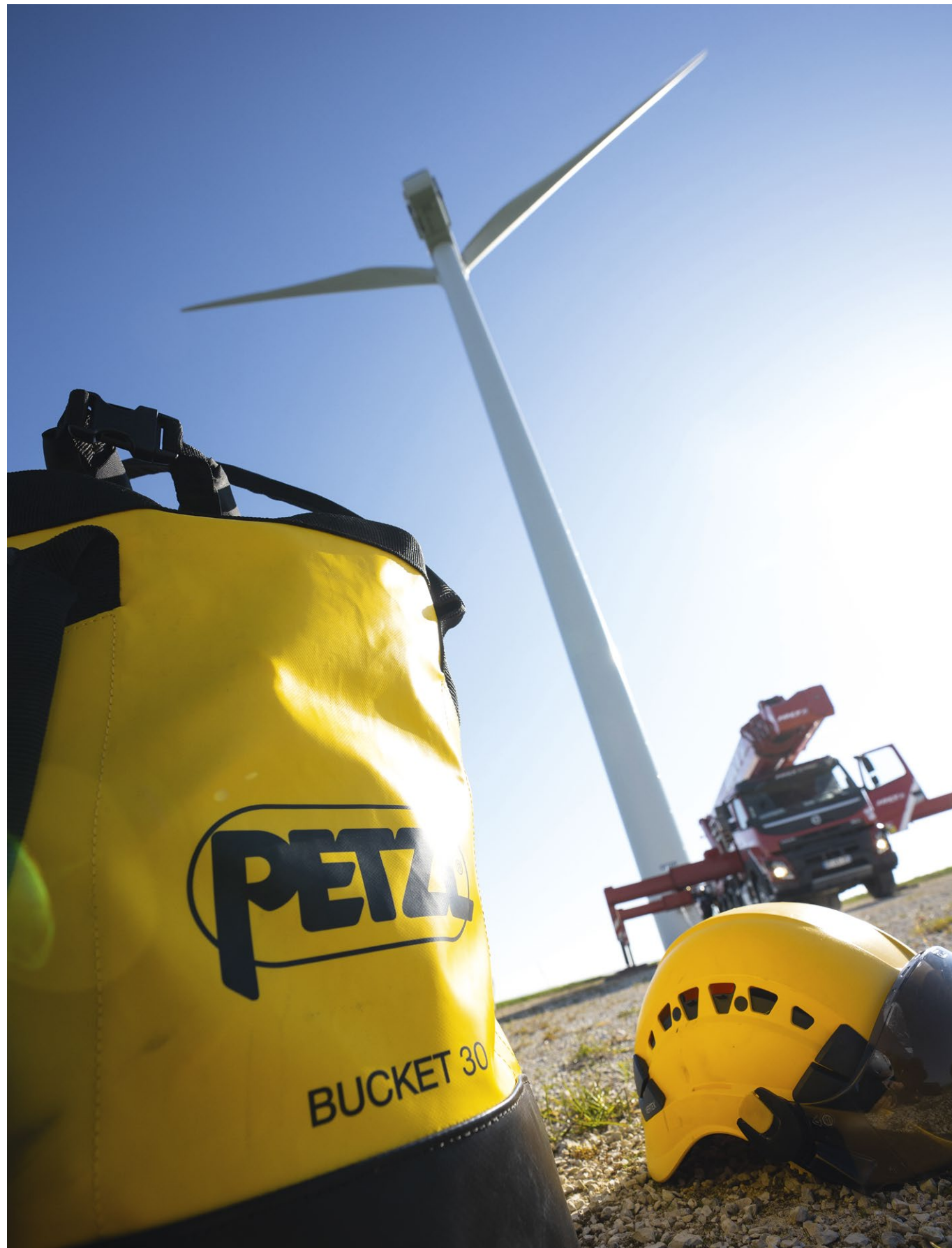
Wind turbine maintenance © 2022 Petzl Distribution - Vuedici.org - GR Wind - Vestas - Joly - EDF Renewables - Les Coteaux wind farm
